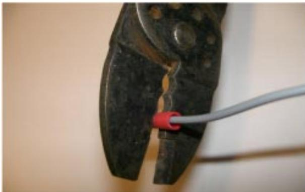
Wire has been pushed in and crimped.
